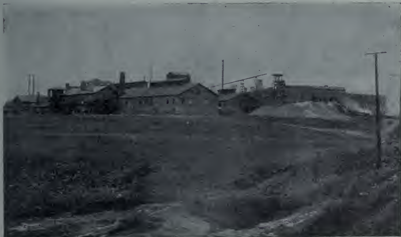
Reduction Mill of Standard Chemical Co., Canonsburg, Pa.
