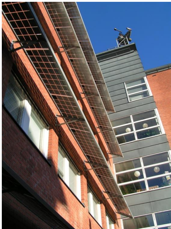
Figure 1 Solar shading installation on Ekologihuset in Lund (architect: M. Pusterla, Fojab; contractors: Switchpower, Gaia Solar; image: M. van Noord)
