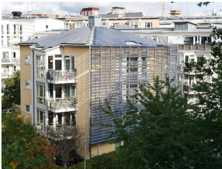
Figure 3 BIPV louvres in Hammarby Sjöstad, Stockholm (contractor: Gaia Solar; image: M. van Noord).
