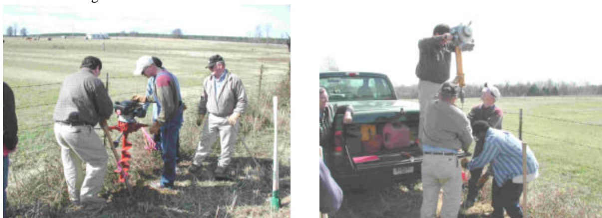
Figure 8-10. Setting deep-driven benchmarks (Memphis District & 3001, Inc.)
