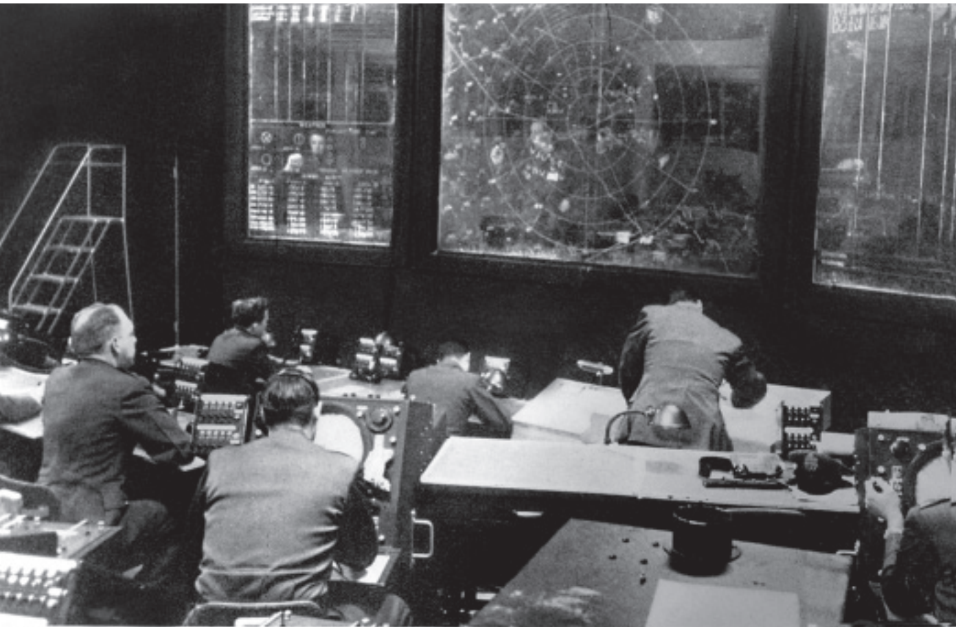
RAND constructed a laboratory replica of an air defense center to study the design, training, and operation of complex human-machine systems.
